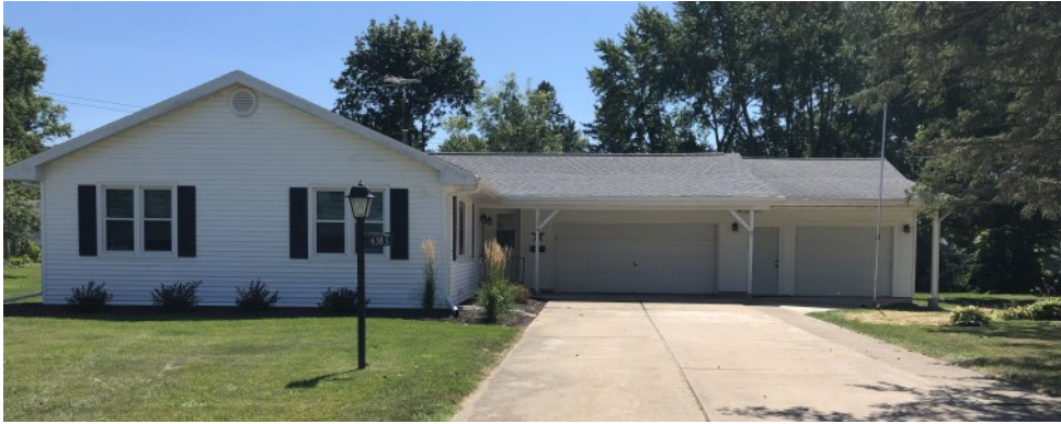
One of our newly renovated residential CILA homes, pictured here, will be opening in September. A second home will open later this fall.
